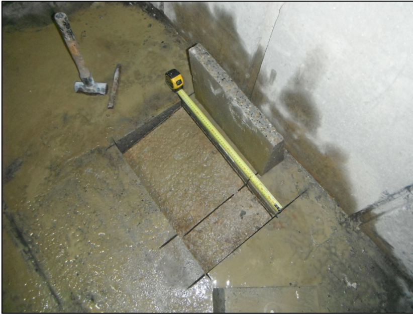
Figure 15: Location of Core/Saw 603. Note apparent footing below initial thin slab
